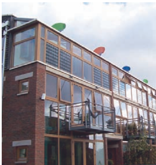
BEDZED housing development, South London showing sunspaces (Architect: Bill Dunster Architects).
