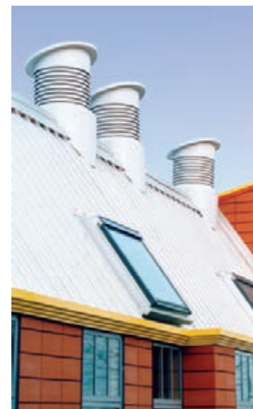
Example of a wind ventilator that catches the prevailing wind for use as natural ventilation, courtesy of Monodraught.
